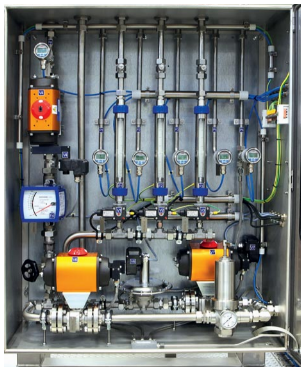
Flottweg Control Unit for the purging and blanketing with inert gas
