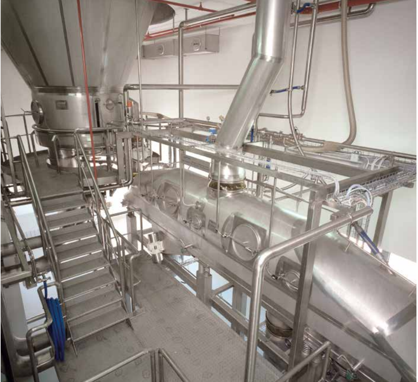
Fluid beds are often used in combination with spray drying plants as an integrated fluid bed or as a separate external fluid bed. The advantages are better product quality and a more efficient drying operation.
