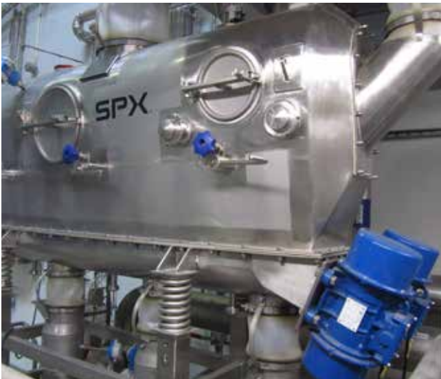
A pilot installation
