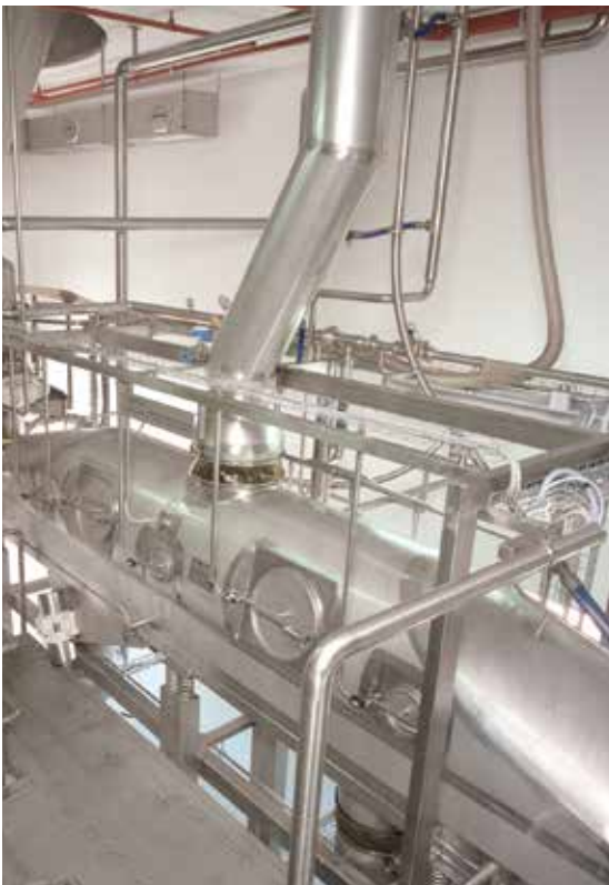
Fluid bed installation
